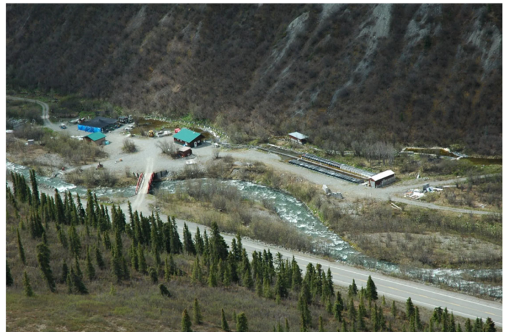
Photo 7. Gulkana Hatchery near Paxson, Alaska.
